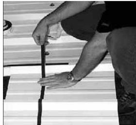
**NEVER USE NAILS** to fasten SunSky panels. The use of nails can damage the panel at the fastening point. Using nails will also prevent the panel from properly expanding and contracting with temperature change, thus resulting in buckling.
